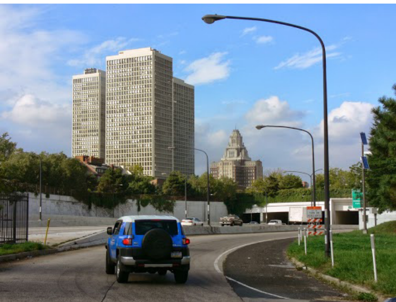
A car entering the Lombard Circle ramp to I-95. The ramp runs a mile and a tenth north through the entire Penn's Landing area, until it discharges onto I-95 just south of the Benjamin Franklin Bridge.
